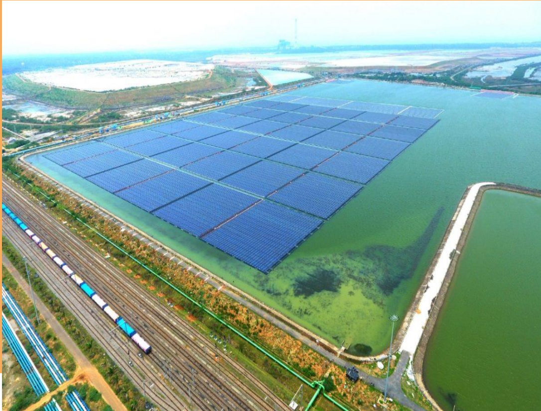
Ramagundam Floating Solar : Capacity Supplied 62 MW.
